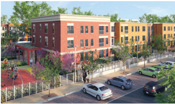
Above: All 504 affordable units at the severely deteriorated Grove Parc will be torn down. An equivalent number of subsidies for low-income renters will be available either on-site in the new development or at other existing buildings in the neighborhood.
